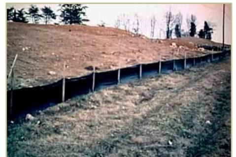
A silt fence can help keep sediment from running into nearby waterways.
