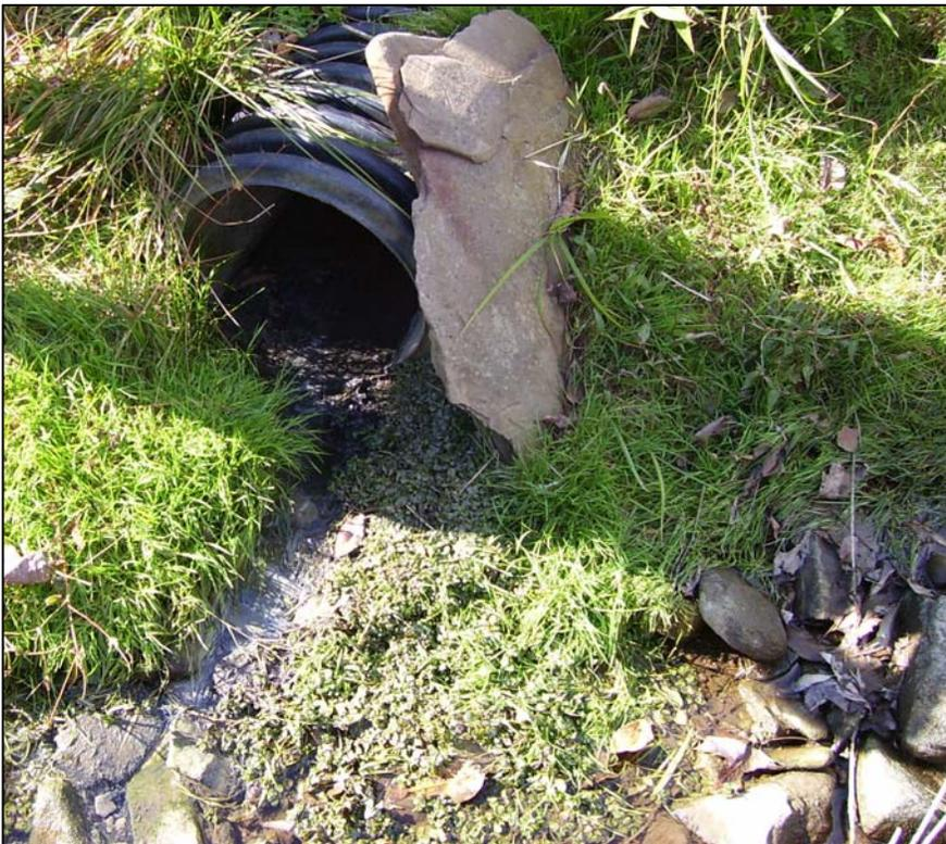
*“Gray water” emerges from a storm sewer outlet near the community of Irondale indicating the presence of sewerage effluent.*
