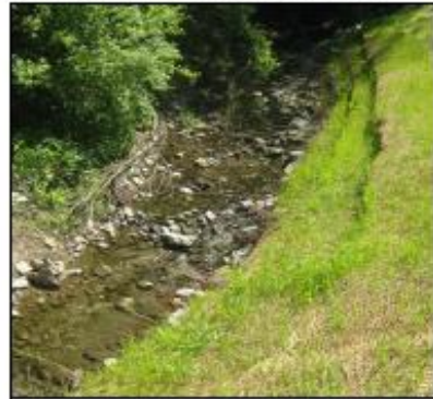
After: JF New & Associates installed three layers of soil lifts
