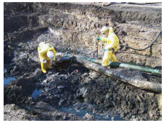
The 2009 Mid-Valley pipeline rupture in northwest Ohio released an estimated 52,000 gallons of crude oil into the Portage River.
