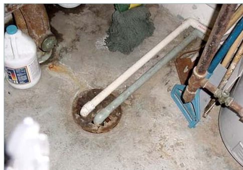
Figure 1. Potential for back-siphonage
