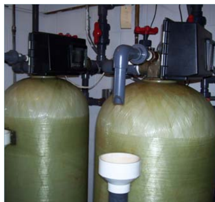
Figure 2. Sufficient air gap
