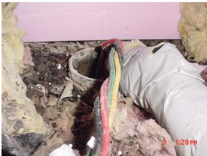
**Lack of a Watertight Cap on a Well**
