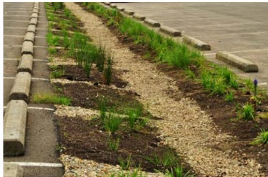
This bioswale/rain garden captures runoff from a large heavily used parking area and diverts it to a vegetated bio-filter. This project was also completed under provisions of BUCK11-01
