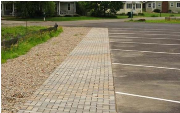
Retrofitting this heavily used boat launch area with pervious pavers and wetland treatment train was completed under provisions of #BUCK11-01.
