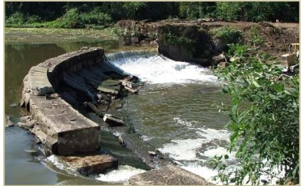
*Serving as both the implementer and borrower, the Summit County Department of Environmental Services used \$1,845,000 in WRRSP funds to complete the Munroe Falls Dam Modification. Successful removal of the 12-foot high Munroe Falls dam restored natural stream flow throughout the area. Accompanying the dam removal was the successful restoration of nearly three miles of streambank as well as stabilization of several tributaries flowing into the former impoundment caused by the dam.*
